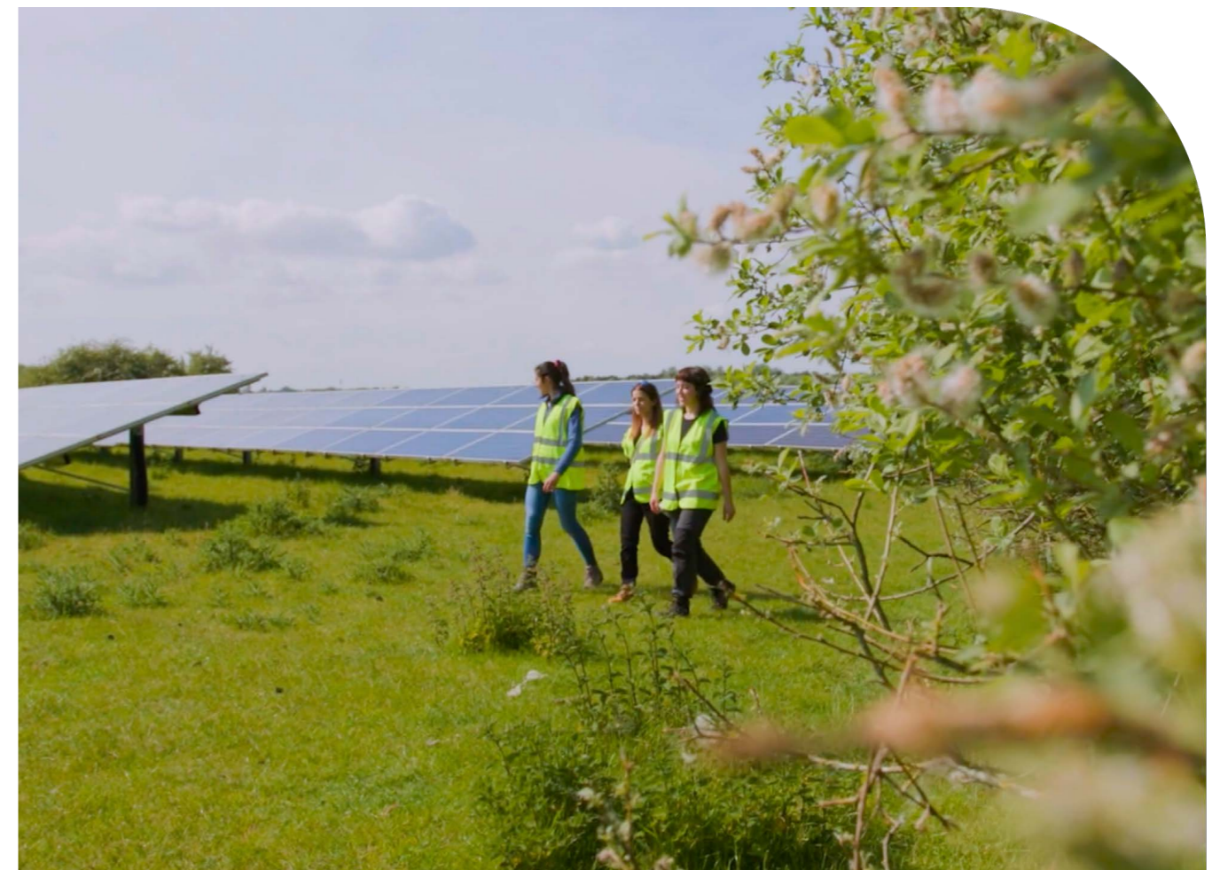
Honington Solar Asset, NextEnergy Solar Fund
